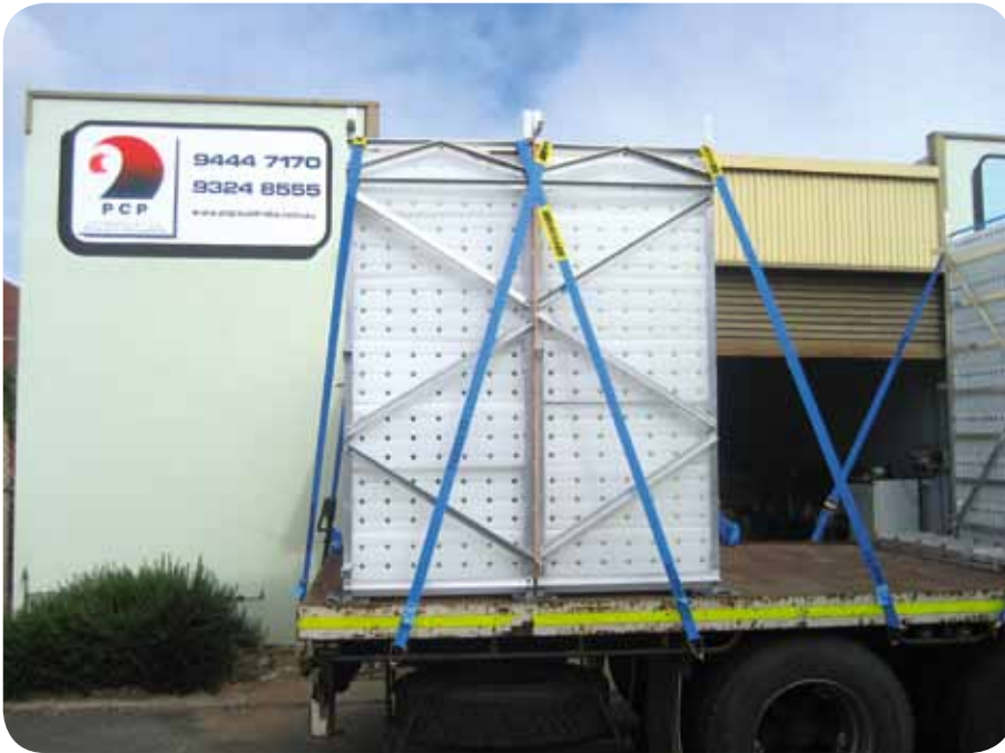
PCM panel installation day.
